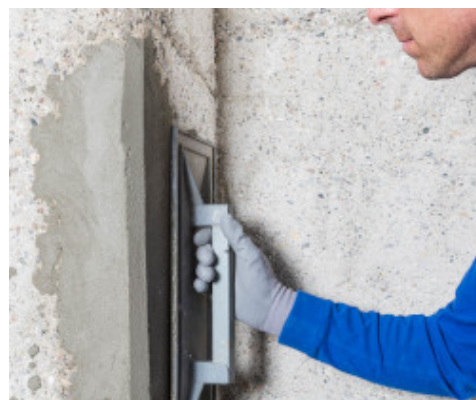
Floating the surface of Planitop Smooth & Repair R4 Zero
