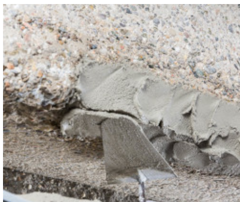
Applying Planitop Smooth & Repair R4 Zero
