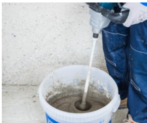
Mixing Planitop Smooth & Repair R4 Zero
